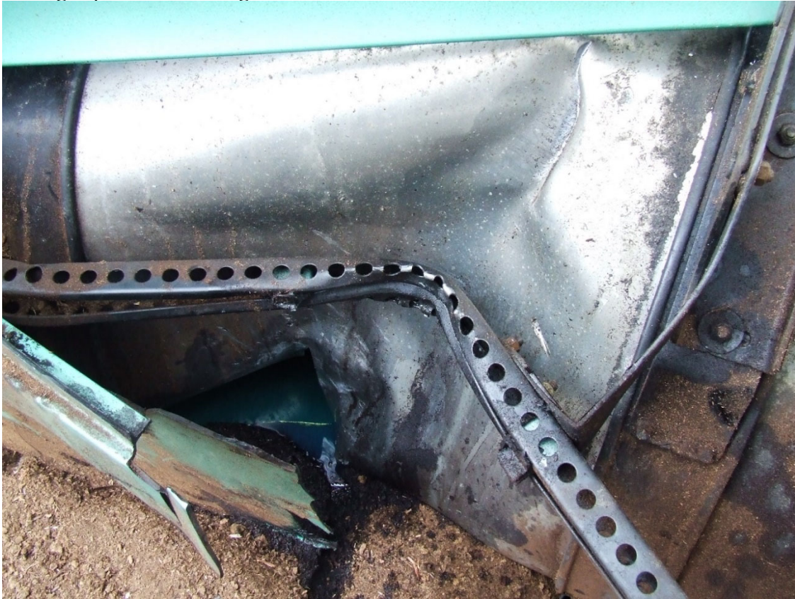
Damaged petroleum storage tank and leak
